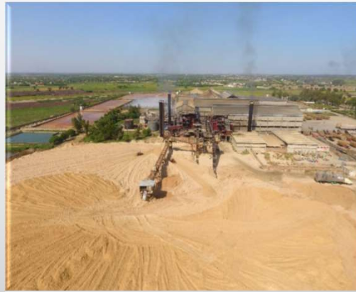
Chashma Unit – 2 Rated Crushing Capacity: 6,000 MT/day
