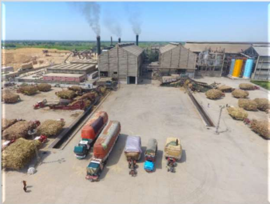
Chashma Unit – 1 Rated Crushing Capacity: 12,000 MT/day
